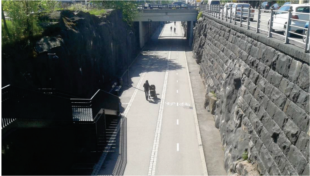
Abb. 5 „Baana Cycleway“ in Helsinki (FIN)
